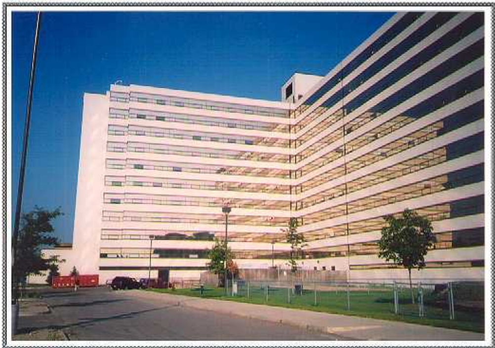
PHOTOGRAPH No. 4 SOUTH SIDE OF THE BUILDING
