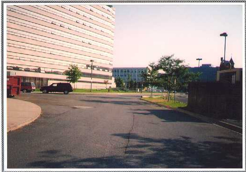
PHOTOGRAPH No. 9 BACK-UP GENERATOR ON RIGHT SIDE OF PHOTO
