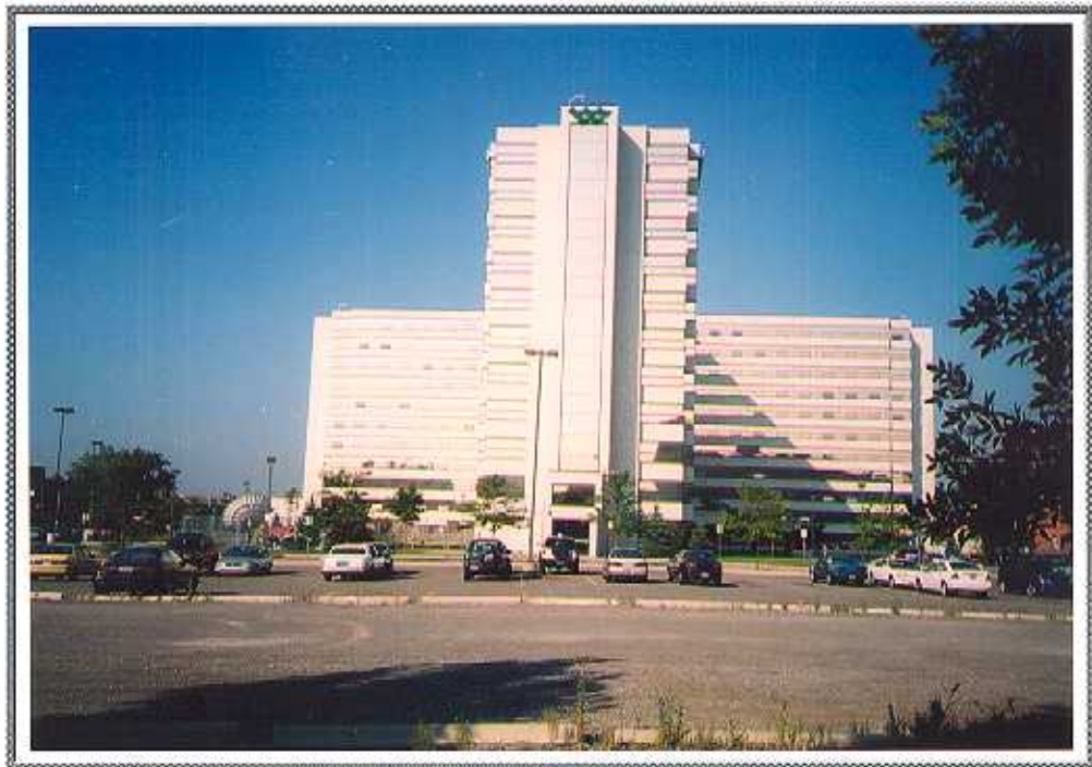
PHOTOGRAPH No. 2 EAST SIDE OF THE BUILDING
