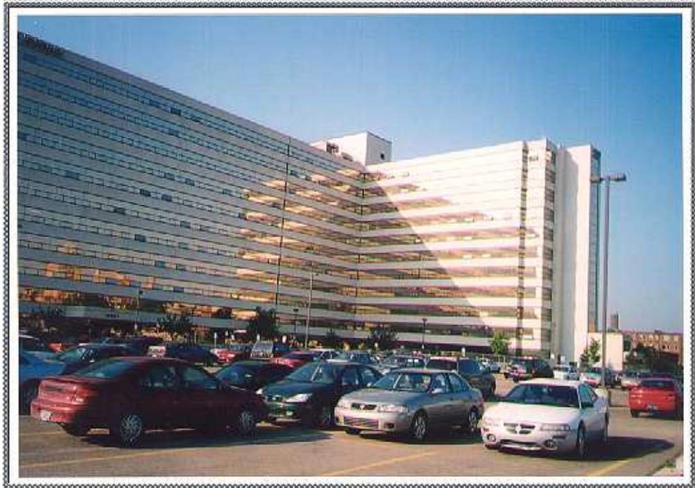
PHOTOGRAPH No. 3 NORTH SIDE OF THE BUILDING
